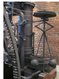
1788: Boulton & Watt's Lap Engine.
