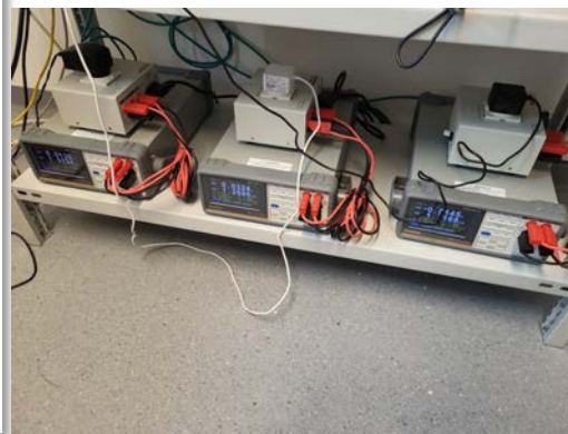
Energy measurement infrastructure
